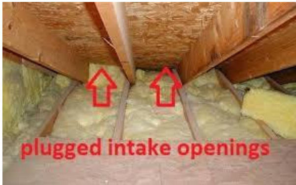
Insulation covering soffit vents
